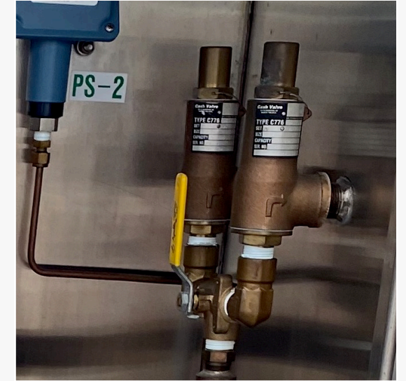
Relief Valve (icing around relief)
