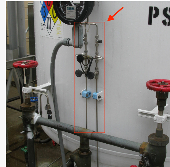
Liquid level gauge lines frosting
